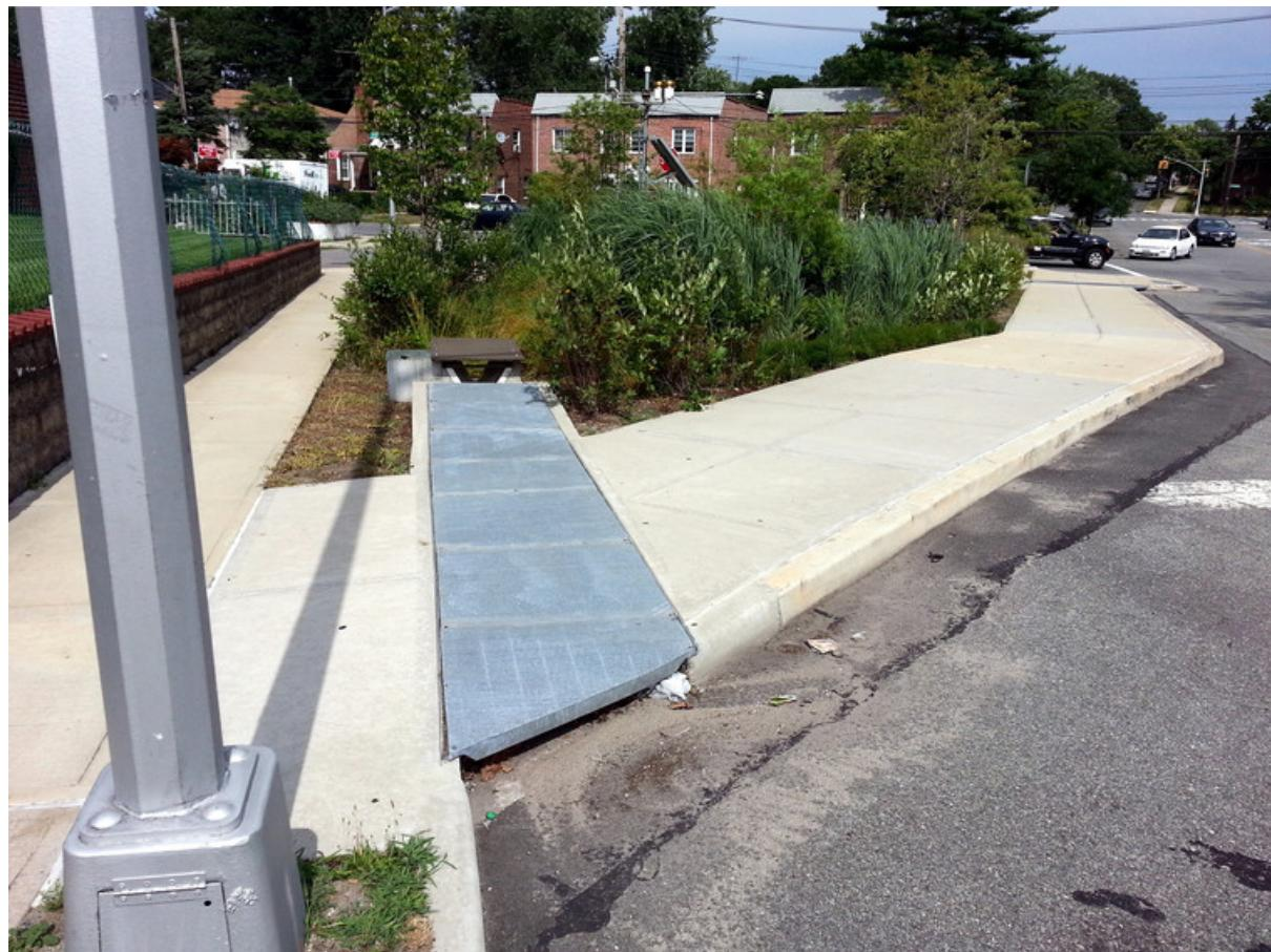
Under New York City's green infrastructure plan, the city has installed 'bioretention facilities' to reduce stormwater runoff and thereby lower the chances of overflow of sewage into local waterways. [imjustwalkin/flickr](#), CC BY-NC-SA
